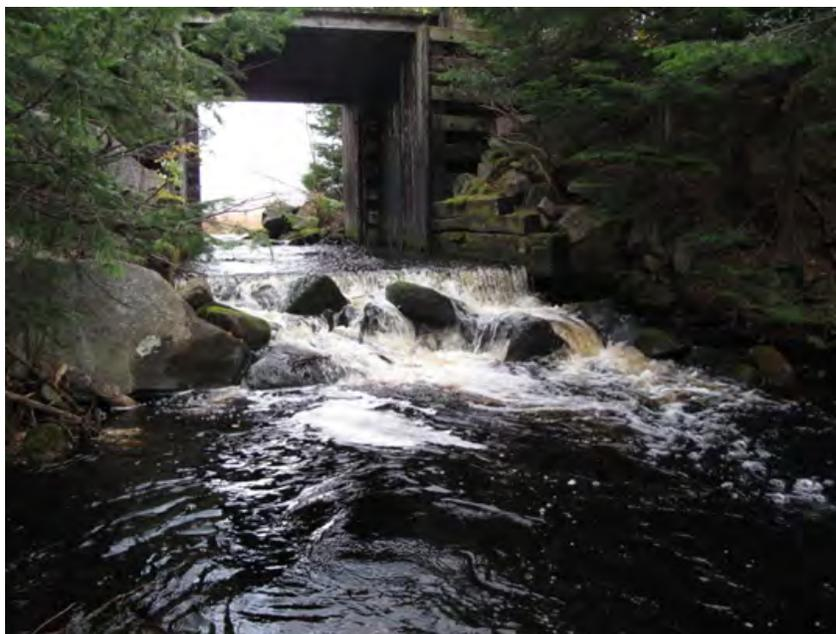
**Figure 5.2 Barrier to Fish Passage Structure at Entrance to Upper Nashwaak Lake.**
